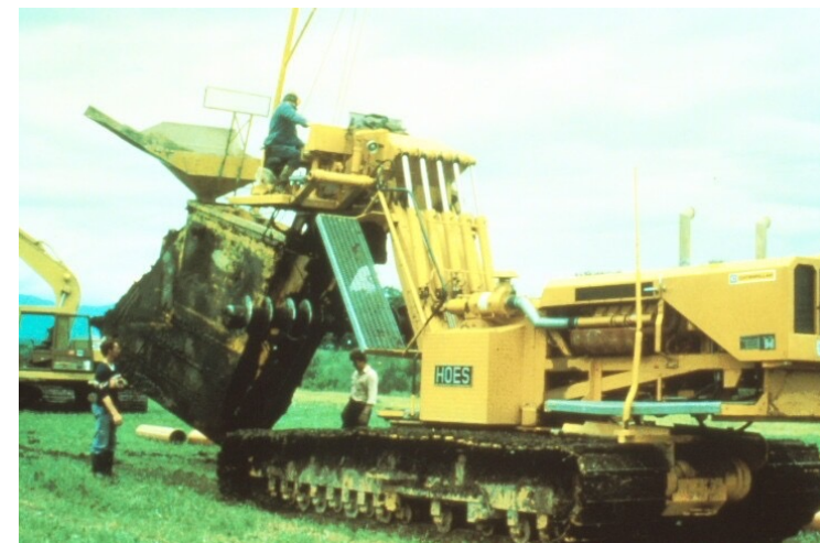
Lecture 13-1. Execution of drainage
